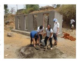
The second group perfected the art of making mud walls as they sang their way through the mixing of sand, cement mud and jaggery water in exact proportions. Much to our delight, the mud that had been pressed into frames was set creating a structure strong enough to withstand the weight of the entire team of students standing on the completed walls at the end of the task.
