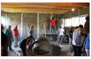
The team continued to work hard in the final phase of the project work at the youth/community centre, plastering the walls with first rough cement and then fine smooth cement and finally buffered it so it was completely ready for painting. They also managed to fit in painting and staining the stage at the major's office which is used for town events and everyone got a certificate of excellence from the major!
