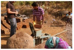
With a team of only 17 students, two leaders, one security, and one DAIS staff member, we had a lot of work to do in very humid conditions. The work to be done on site was mixing concrete, making mud bricks weighing 11 kg each, and made manually with a machine by the team members. These bricks needed to be carried in a chain over the distance of approximately 300m up a hill, this was the work in which took the most amount of people
